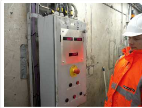
Assessment of (a part of) a bridge control system
