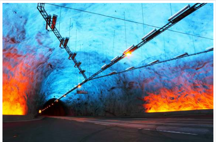
Figure 1: Daylight cave inside the Laredal-tunnel in Norway
